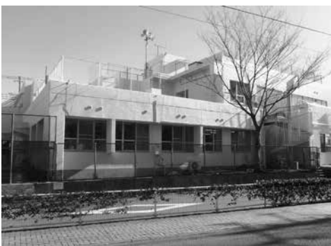
The renovated East Multigenerational Communication Center
